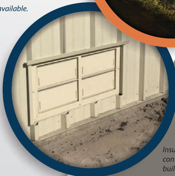
*Insulated Series in 2 x 2 multi-frame configuration, installed in a metal building, powder coated wheat*
