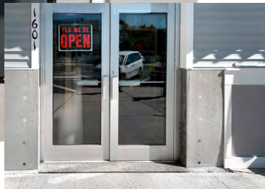
Permanently Installed Wall Anchors
